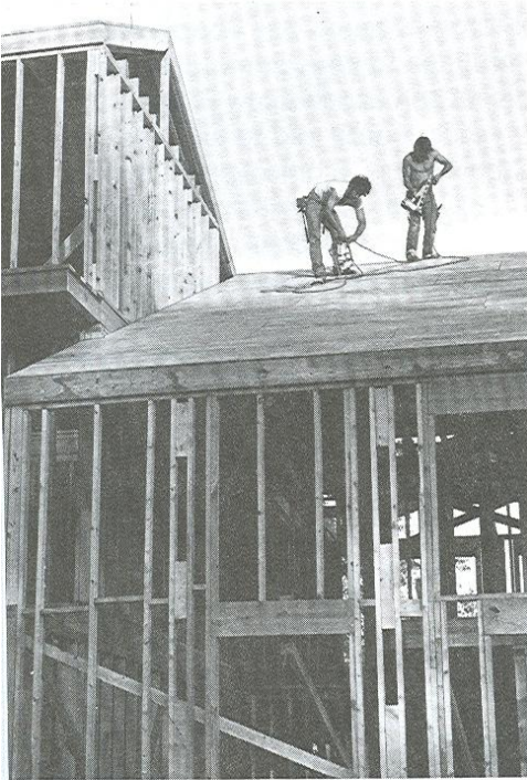
Southern Forest Products Association Figure 5-3. The framework of this building is constructed of softwood lumber.
